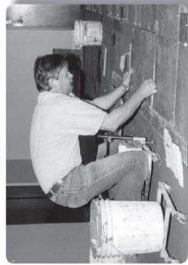
Solution: Laying tile with kneeling creeper
